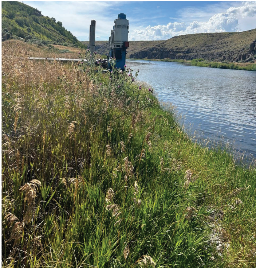
Figure 6. Second angle of pumpstation at Rick's Property POD site. Reed canarygrass densely covers the river margin; higher elevation areas at this site are covered with a mixed community dominated by smooth brome. Photo taken facing downstream.
