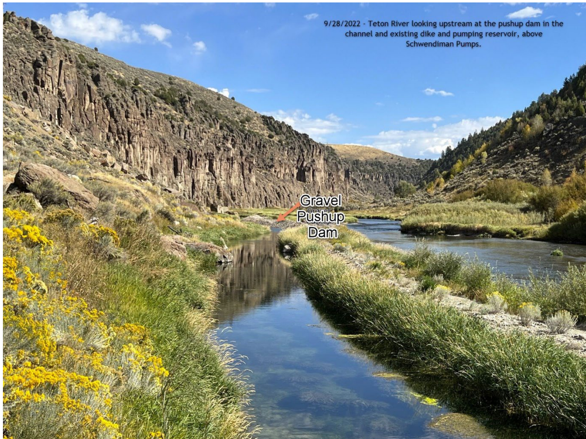
Figure 4. Teton River looking upstream at the rock check structure in the pump channel and existing dike (to be elevated) above Site 1-Schwendiman Irrigation System
