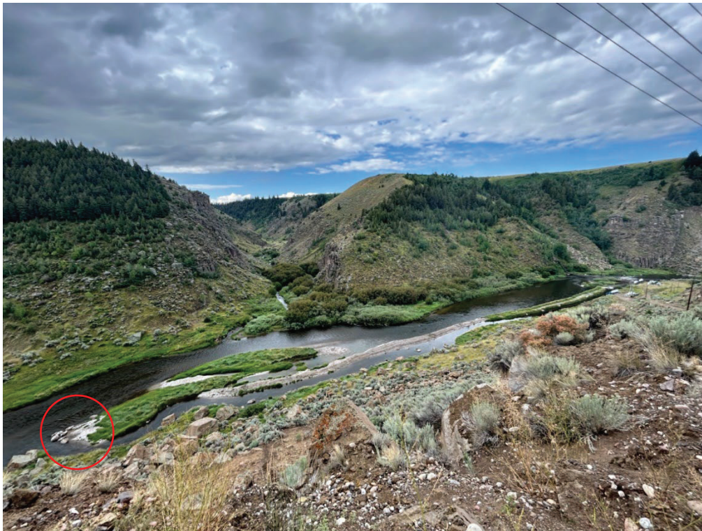
Figure 3. Second view of Schwendiman site from the access road. Pumpstation is visible on the near bank of the Teton River at far right and the entire length of the elevated gravel dike with upstream rock check structure (circled) are visible running diagonally through the photo. The Teton River flows from left to right of this photo.
