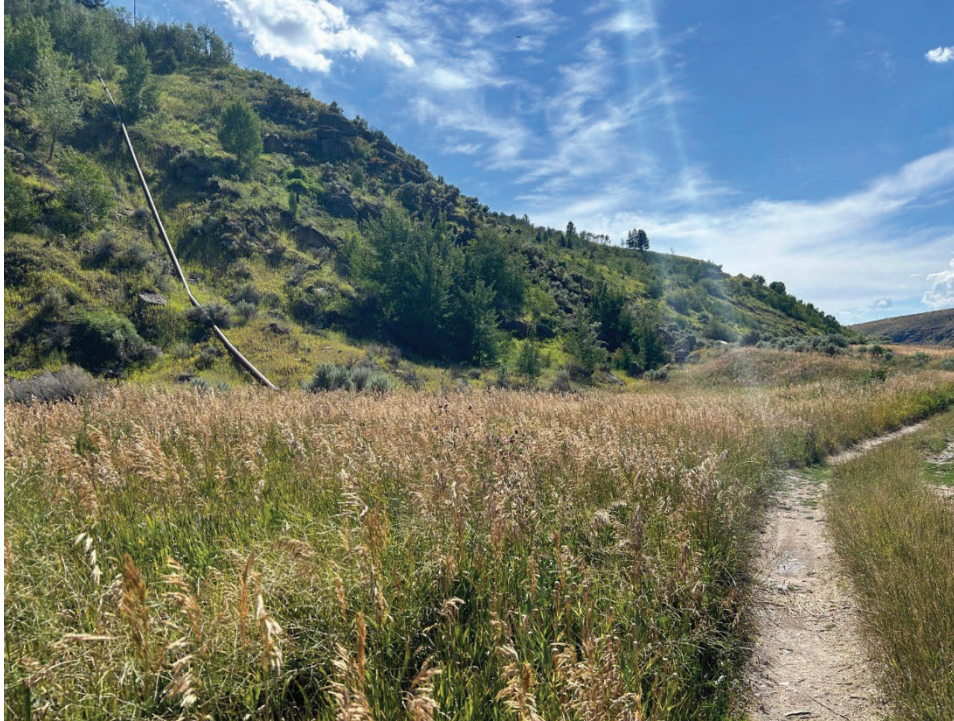
Figure 7. Rick's Property POD site, taken from pumpstation location (to right out of photo frame) and facing downriver. Access road leading to canyon rim is visible at right of photo; main water conveyance pipeline visible at left.
